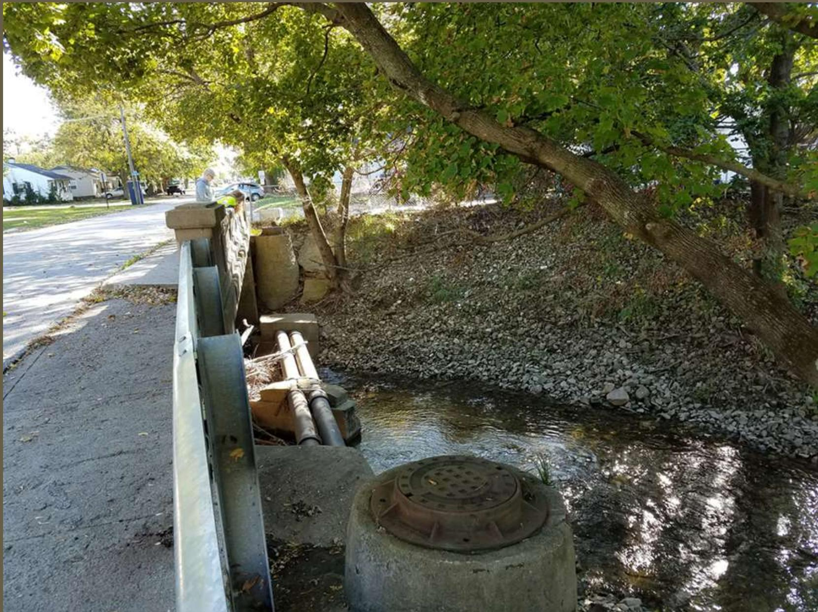
View of the Park Street Bridge taken from north side of bridge. Rock on left bank extends to top of bank. Note debris in the pipes
